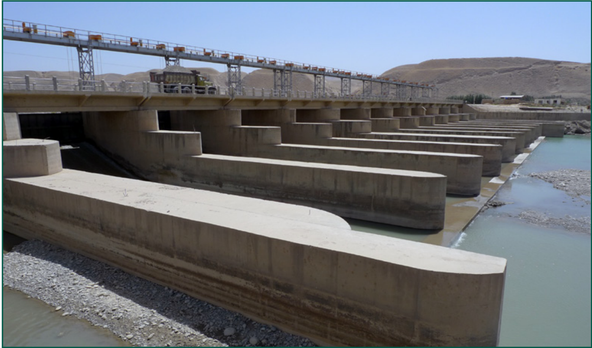
Image 4: Khanabad barrage in August 2011
