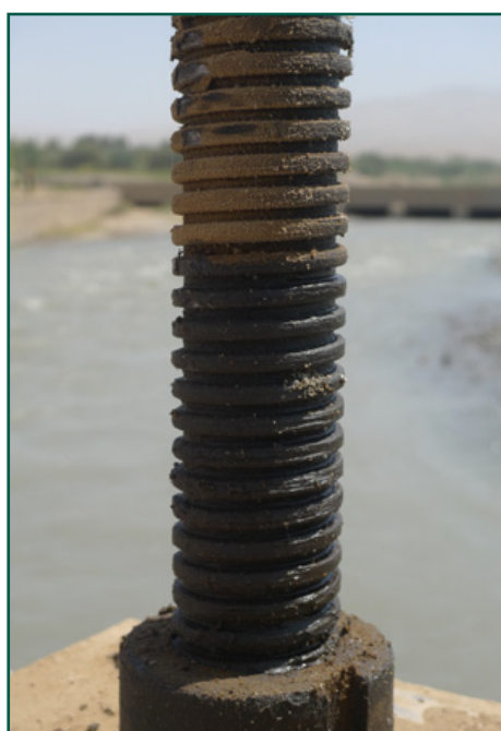
Image 3: The grease on the screw from a Sharawan gate indicating that it has been opened while it should have been kept closed
