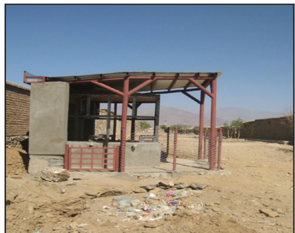
Water kiosk, informal settlement (Charikar)
